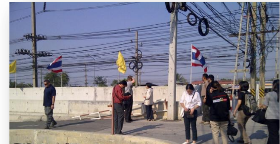
LMI PR DREE IPC participants inspect the Bang Pa-In Industrial Estate flood protection system in Ayutthaya Province.
